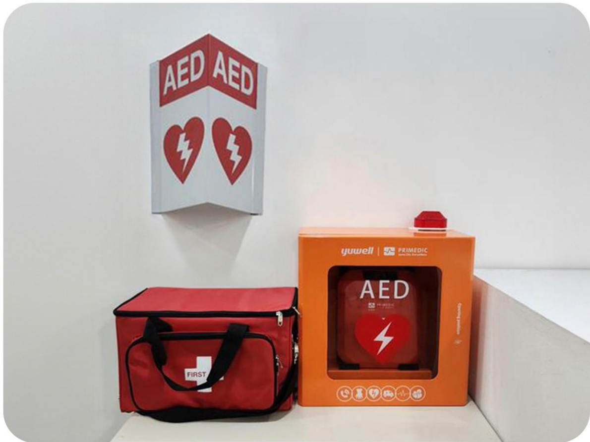
AED and First Aid Kit Installation Project at the Office
